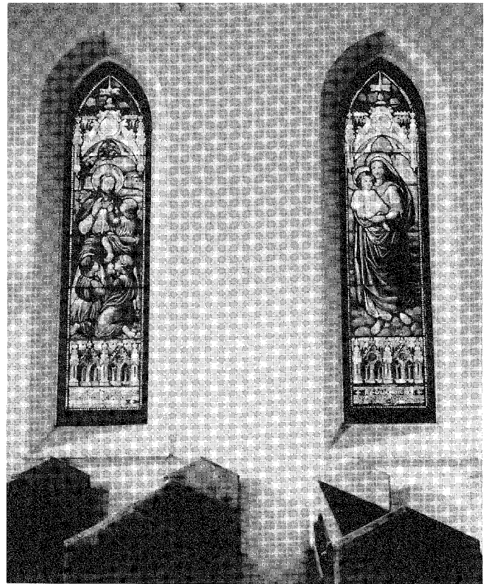
Original lancet windows in the nave have been replaced by stained glass windows with religious figures.
