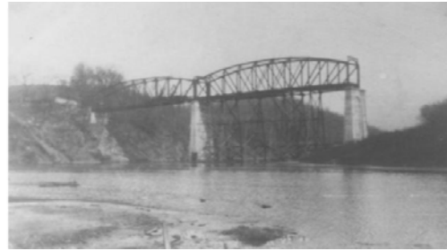
Warren Road Bridge Under Construction c. 1920. (Photo courtesy HSBC collections.)
